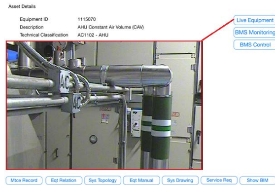
Fig. 6. CCTV live feed in the BIM-AM system at the mobile terminal
